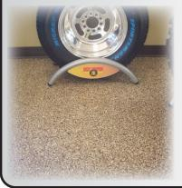
Polyaspartic floors are a multi-coat chip (flake) broadcast coating system. It is designed to provide a capable, seamless flooring finish suitable for numerous types of commercial and residential flooring applications, including garage floors.
